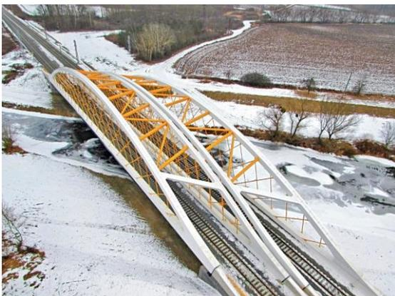
The reconstruction consisted in the removal of a technically unsuitable bridge at km 80,930 of the railway line and provision of the requested railway line speed of 160 km/hour. The original three consecutive structures were replaced with a bridge with a single opening, as requested by the Morava River Basin Agency.
