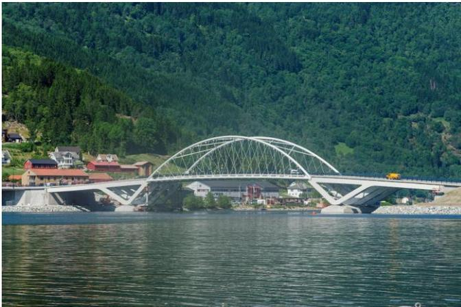
Loftesnesbrui is a 194-meter-long steel bridge, situated in the town of Sogndal by the Sognefjord. The bridge has a network tied arc in the main span, and the middle of the arc is 15 meters high, from top to bottom. The new Loftesnesbrui bridge was built because the old bridge over the Loftesnes sound was very narrow, and it was starting to show signs of wear and tear. The bridge from 1958 had almost no space for pedestrians.
