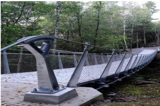
The bridge is in the Groruddal area, linking the city centre with the recreational areas east of Oslo. The Jungle bridge lifts the pedestrians up into the trees, respecting the untouched valley below. It is a simple suspension bridge over a small river, maximizing the use of prefabricated lightweight elements. Elements are hot-dip galvanized for corrosion protection.
